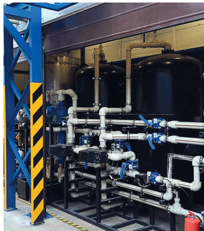
HURIKAN 1000 R - oil sludge disposal
